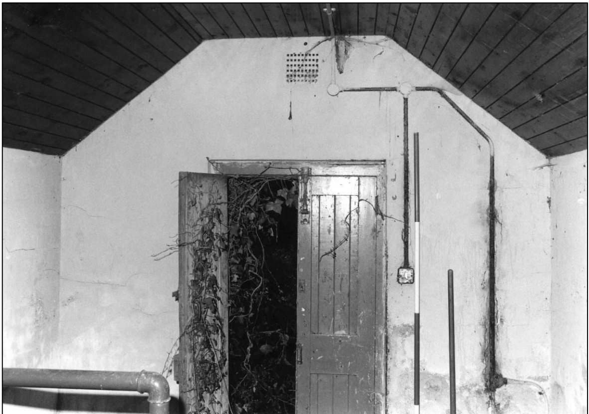
Plate 10: Interior of pump house, looking W (photo 9/12).
