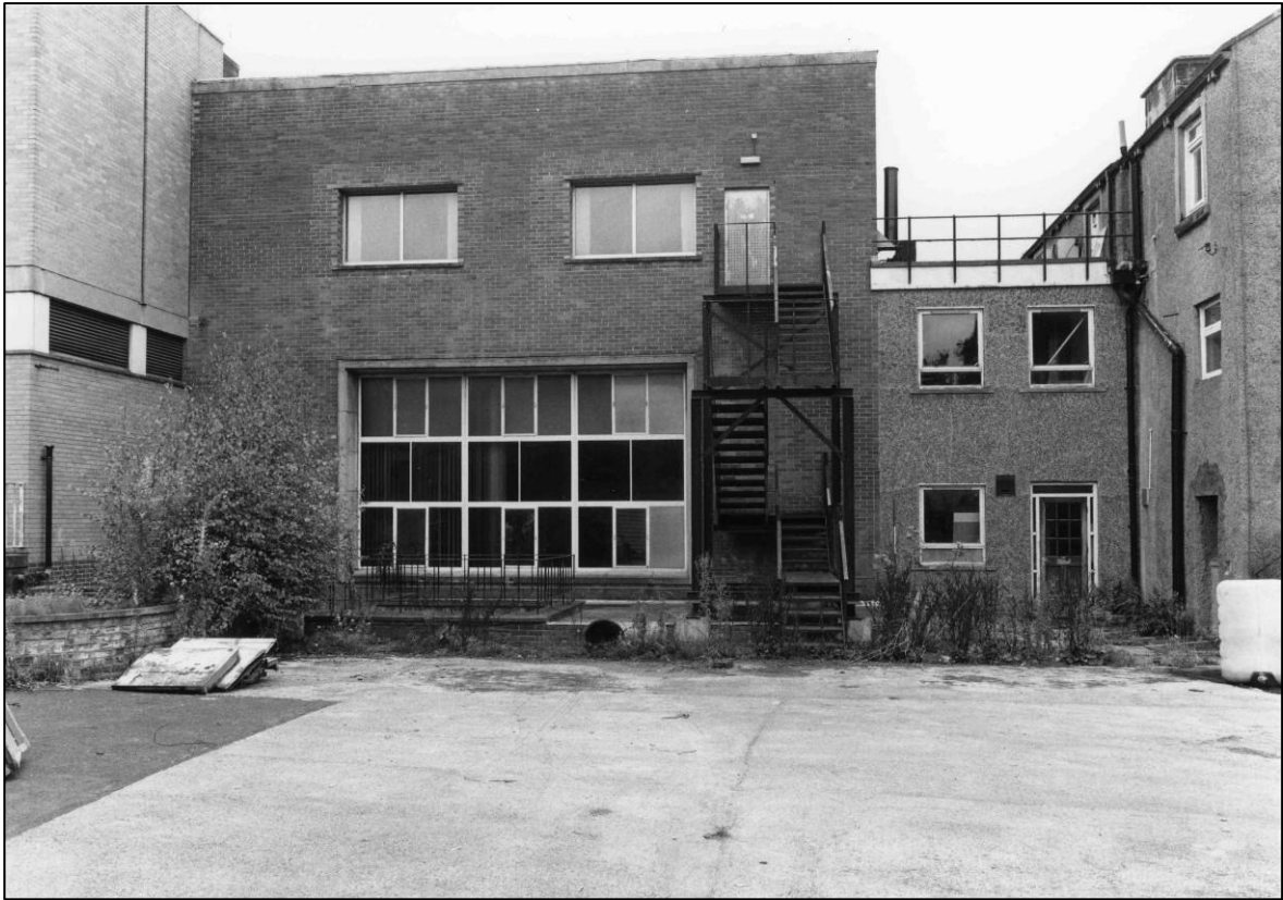
Plate 37: Control Centre complex, S end of W elevation, looking NE (photo 8/15).
