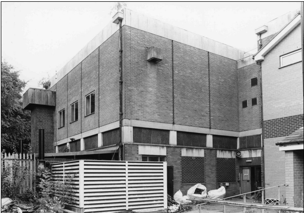
Plate 30: Control Centre complex, N end of W elevation, looking N (photo 8/10).
