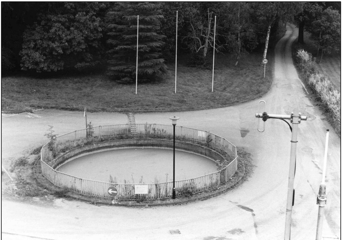
Plate 4: Fire hydrant pond, looking NE (photo 9/6).
