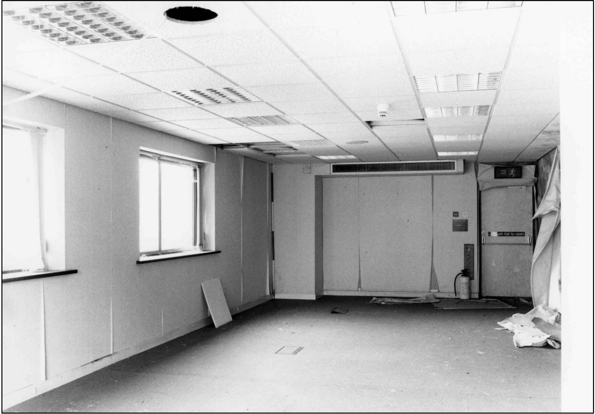
Plate 117: Room 2F1, looking NE (photo 2/15).
