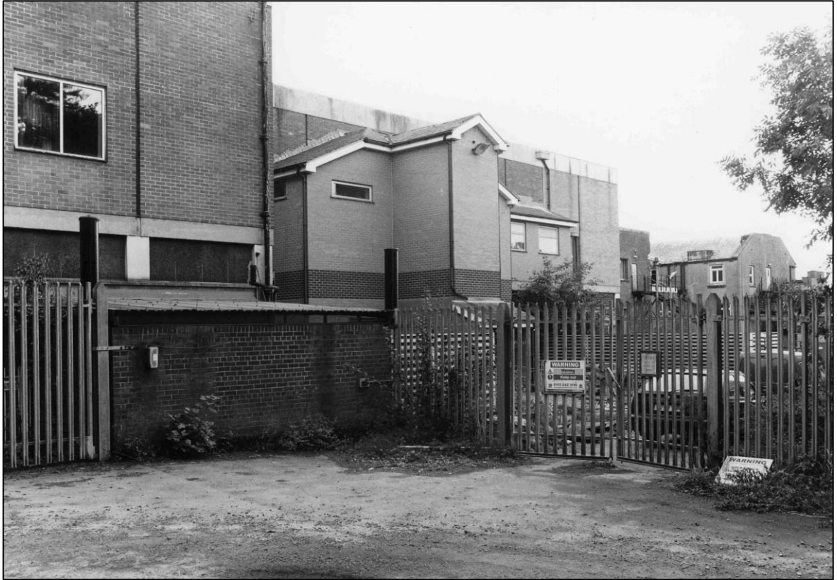
Plate 31: Control Centre complex, central part and N end of W elevation, looking SE (photo 8/9).
