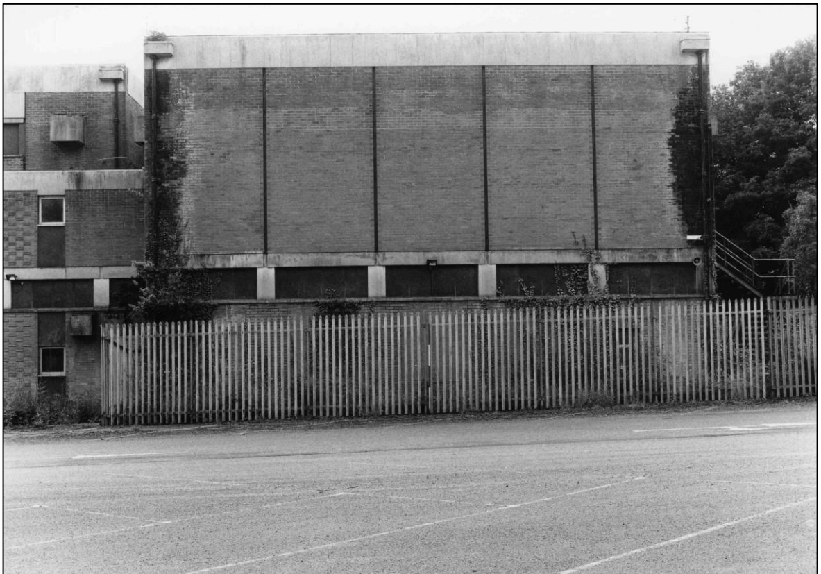
Plate 22: Control Centre complex, N end of E elevation, looking SW (photo 7/15).
