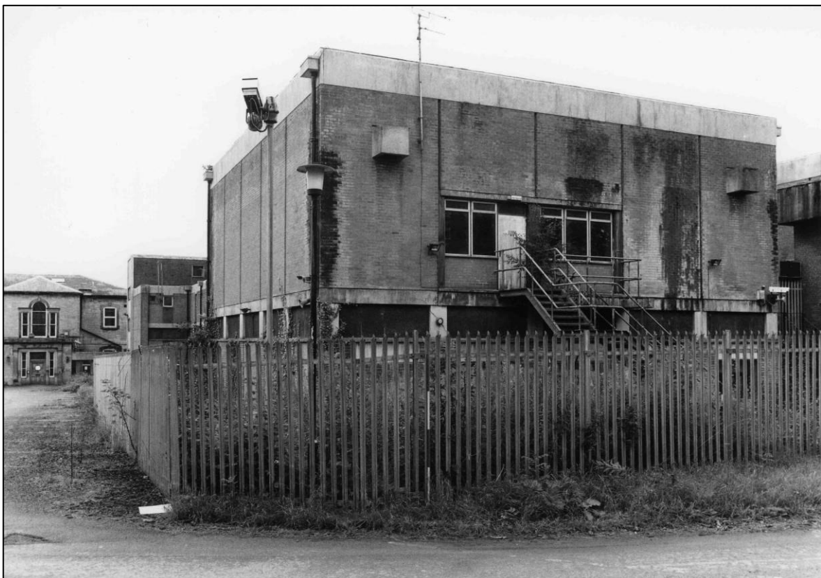
Plate 24: Control Centre complex, E end of N elevation, looking SE (photo 7/17).
