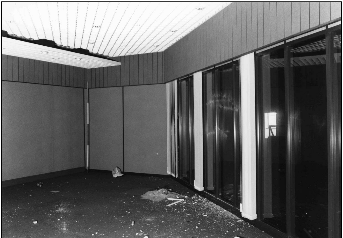
Plate 82: Viewing gallery (1F4), looking SW (photo 2/1).
