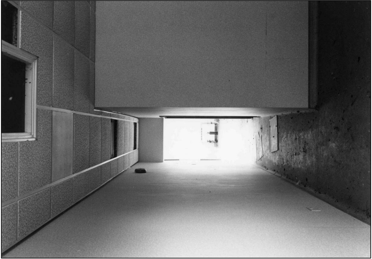
Plate 101: Corridor 1F17 and Mess Room (1F18), looking SE (photo 3/13) (top to left).
