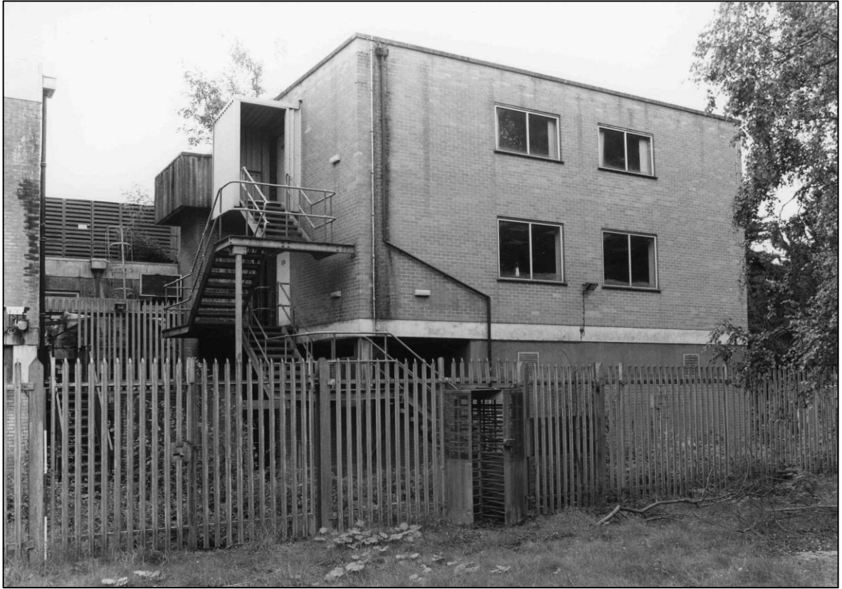
Plate 27: Control Centre complex, W end of N elevation, looking S (photo 8/3).
