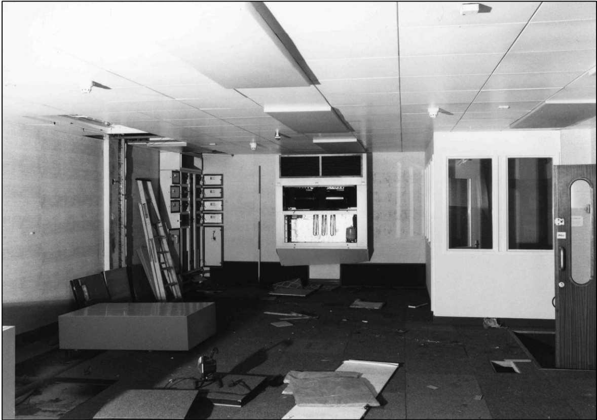
Plate 59: Apparatus Room 5 (GF22), looking SW (photo 5/4).
