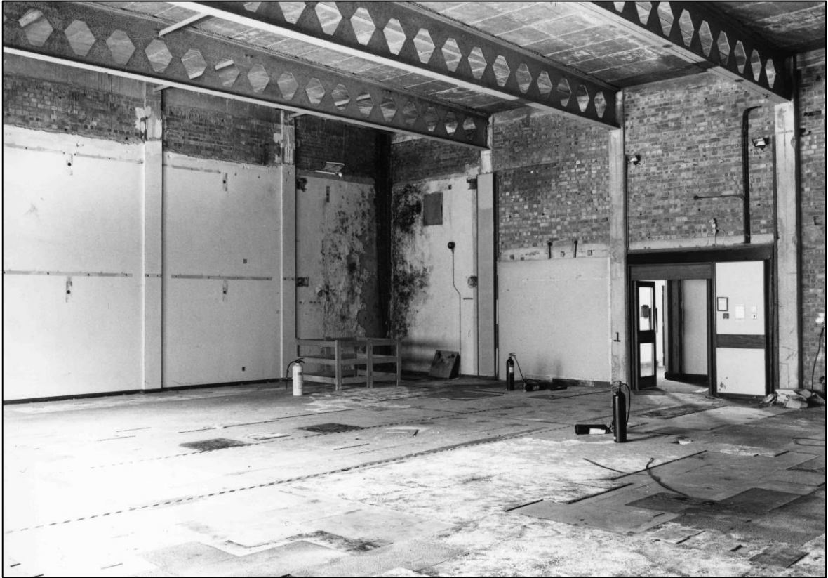
Plate 115: Interim Control Room (1F25), looking E (photo 3/4).
