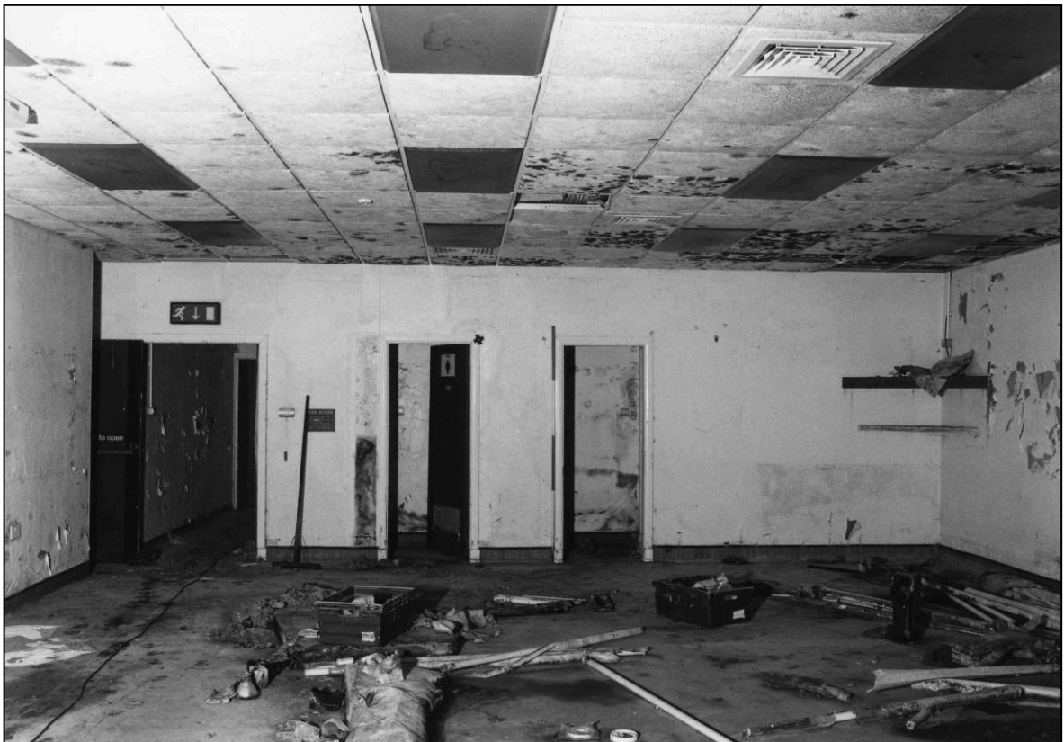
Plate 42: Former Apparatus Room 1 (B10), looking SW (photo 6/2).
