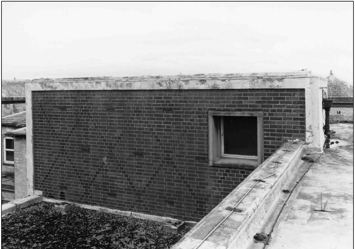
Plate 14: Control Centre complex, uppermost N external elevation of stair tower at S end of E elevation, looking E (photo 9/5).
