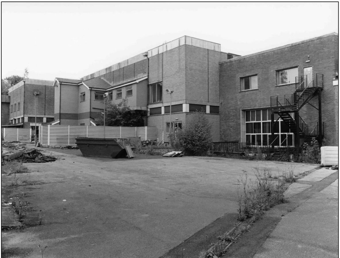
Plate 34: Control Centre complex, central and S parts of W elevation, looking N (photo 8/13).
