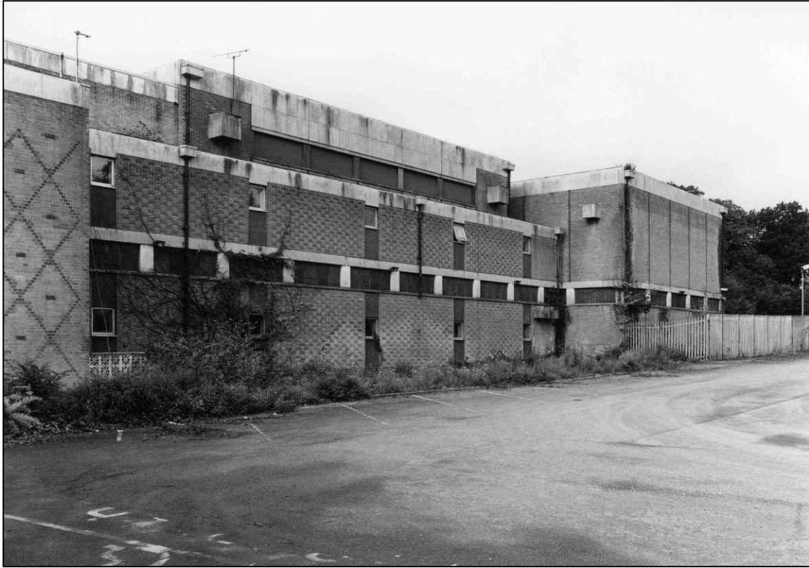
Plate 19: Control Centre complex, central part and N end of E elevation, looking W (photo 7/11).
