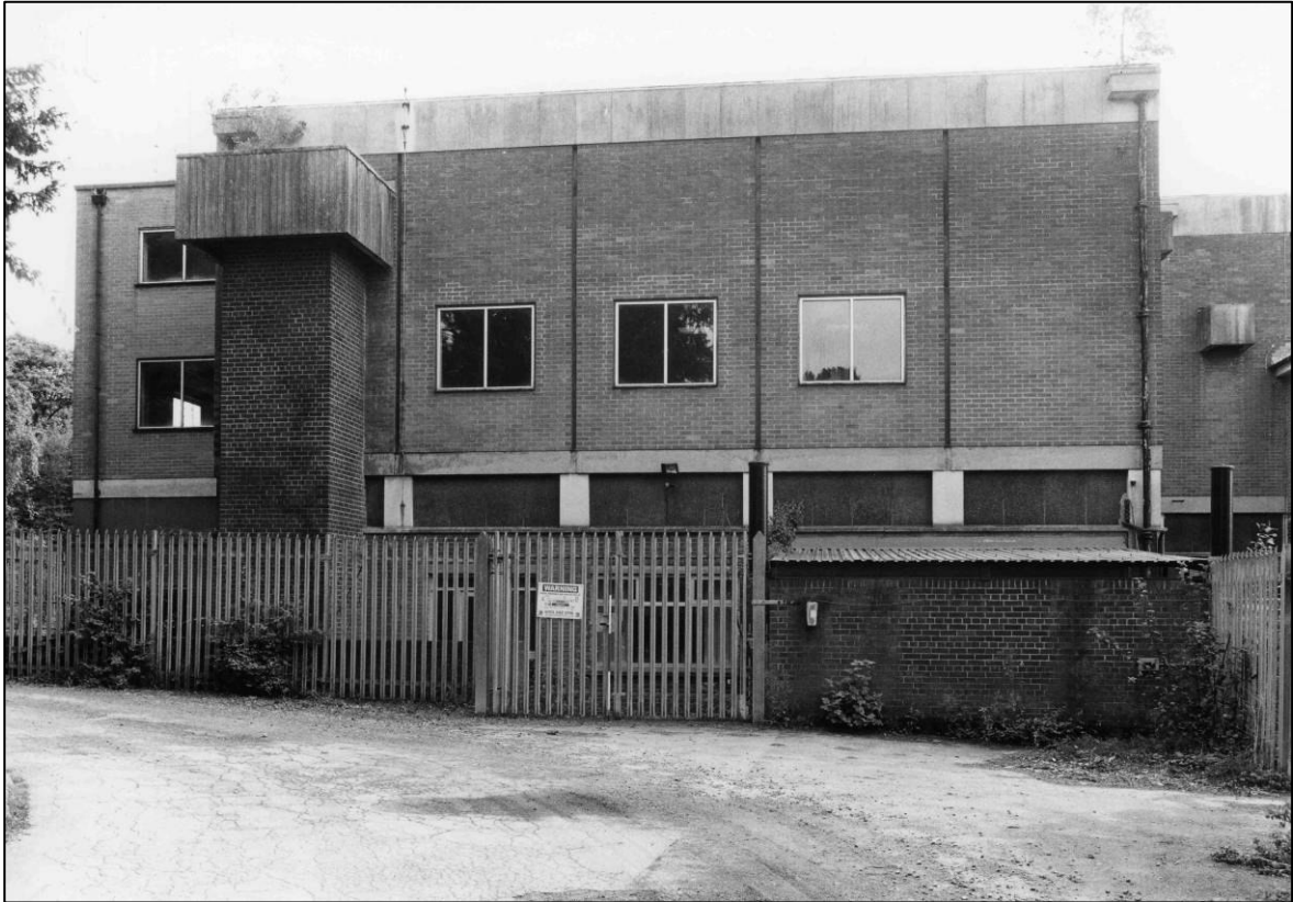
Plate 29: Control Centre complex, N end of W elevation, looking NE (photo 8/7).
