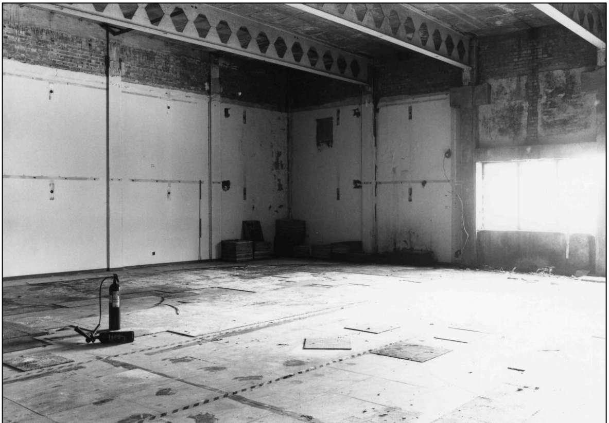
Plate 110: Interim Control Room (1F25), looking W (photo 3/6).
