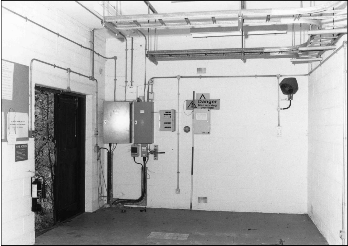
Plate 7: Interior of radio building, looking W (photo 9/10).
