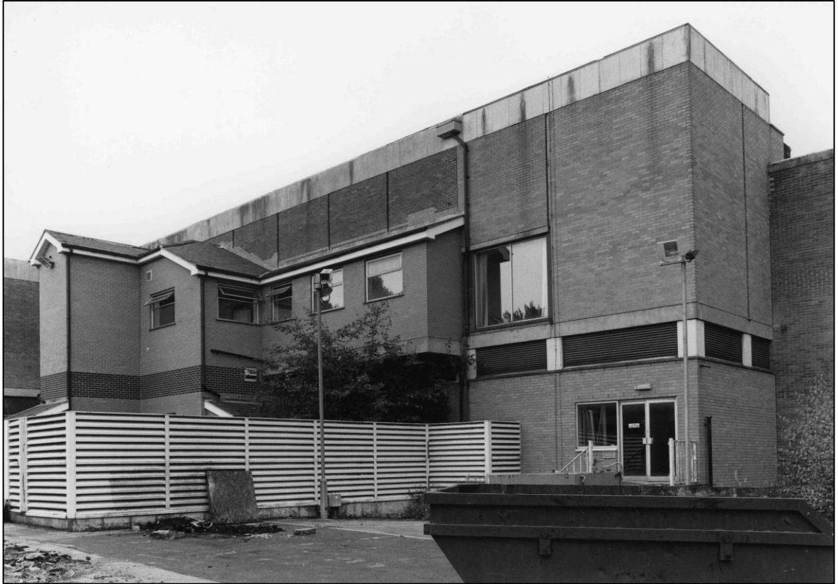
Plate 33: Control Centre complex, central part of W elevation, looking N (photo 8/12).
