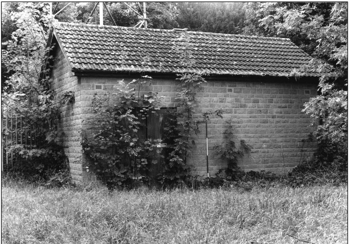
Plate 6: Radio mast building, looking N (photo 8/5).
