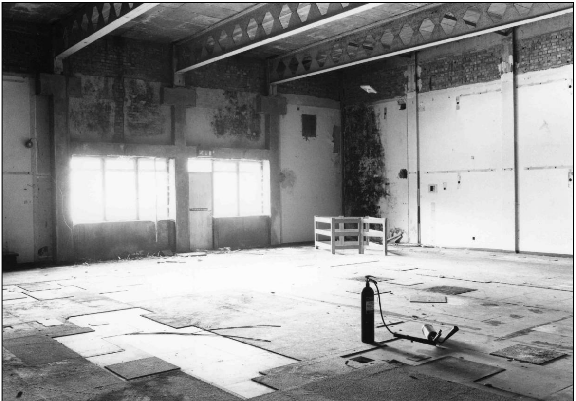
Plate 113: Interim Control Room (1F25), looking N (photo 3/5).
