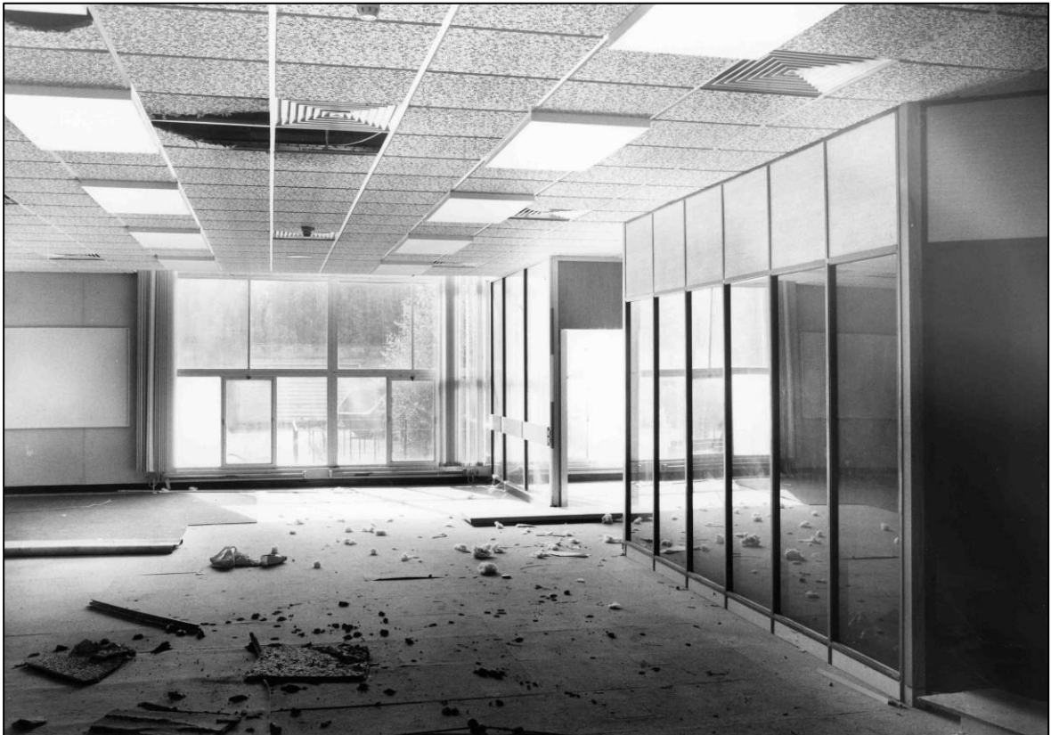
Plate 50: Former East Coast District Control Room (GF1), looking SW (photo 4/12).
