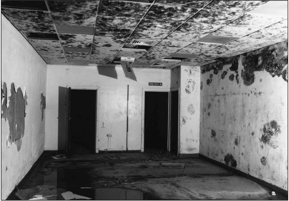
Plate 43: Former Apparatus Room 1 (B11), looking SW (photo 6/4).
