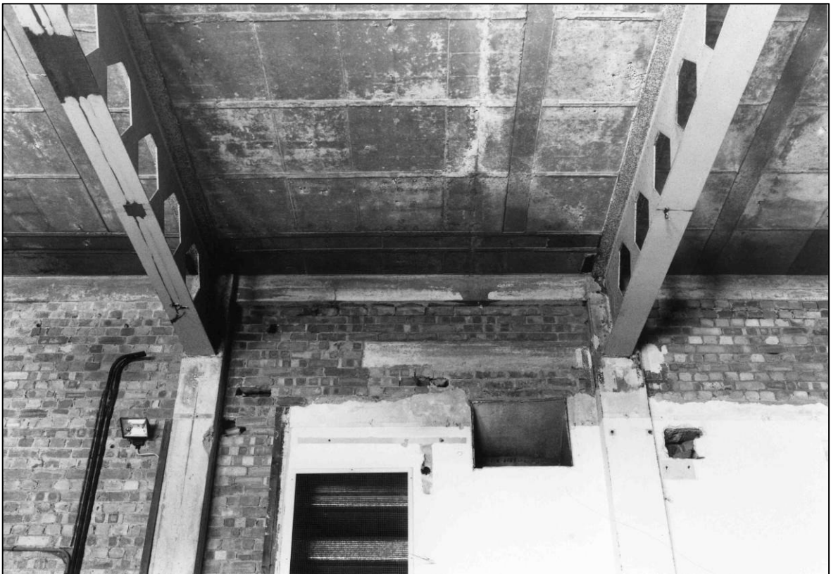
Plate 112: Interim Control Room (1F25), concrete frame and girders to S wall, looking SE (photo 3/12).
