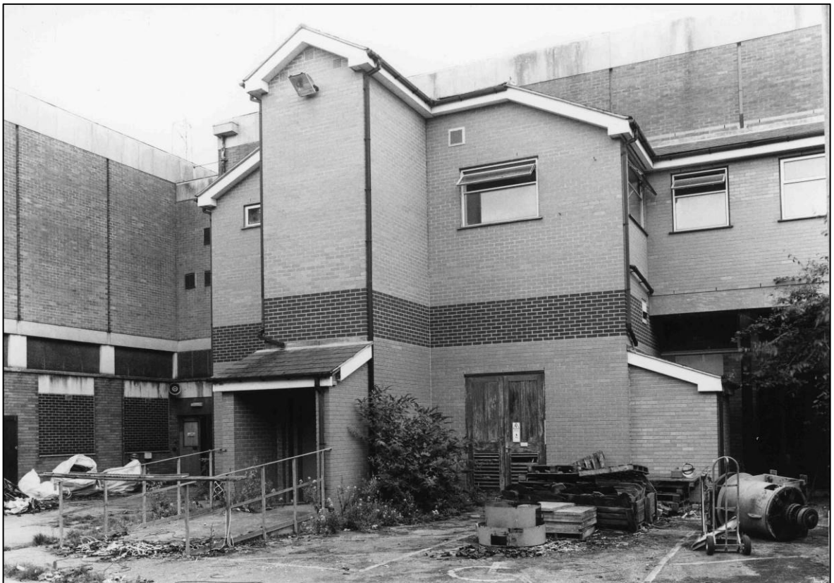
Plate 32: Control Centre complex, central part of W elevation, looking N (photo 8/11).
