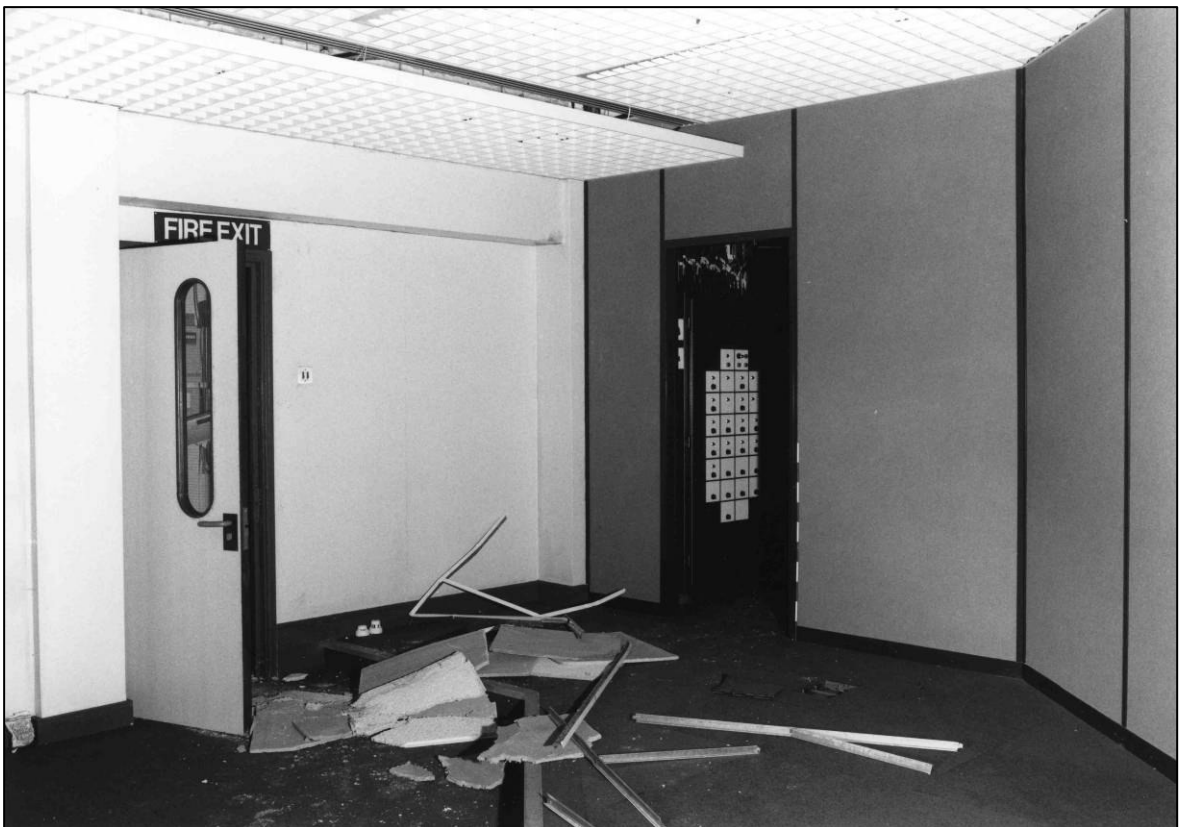
Plate 98: Triangular office (1F16), looking NE (photo 2/10).
