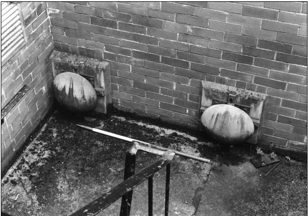
Plate 36: Stairway B1, covered openings in S wall, looking SE (photo 9/2).
