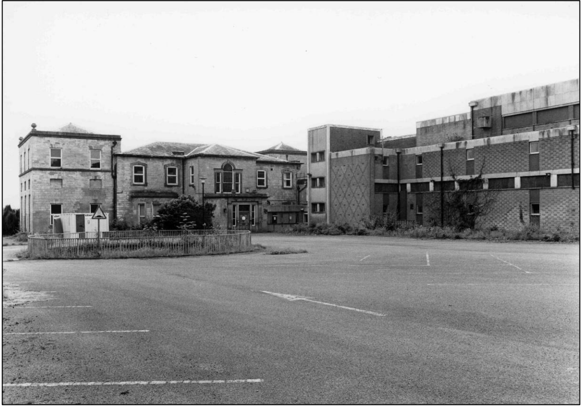
Plate 1: Becca Hall and Control Centre complex, looking S (photo 7/1).
