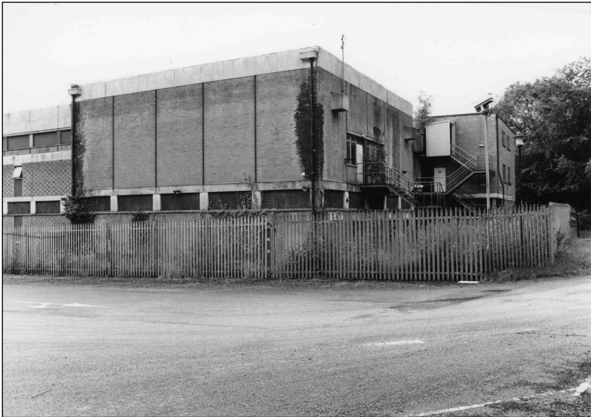
Plate 23: Control Centre complex, NE corner, looking S (photo 7/16).
