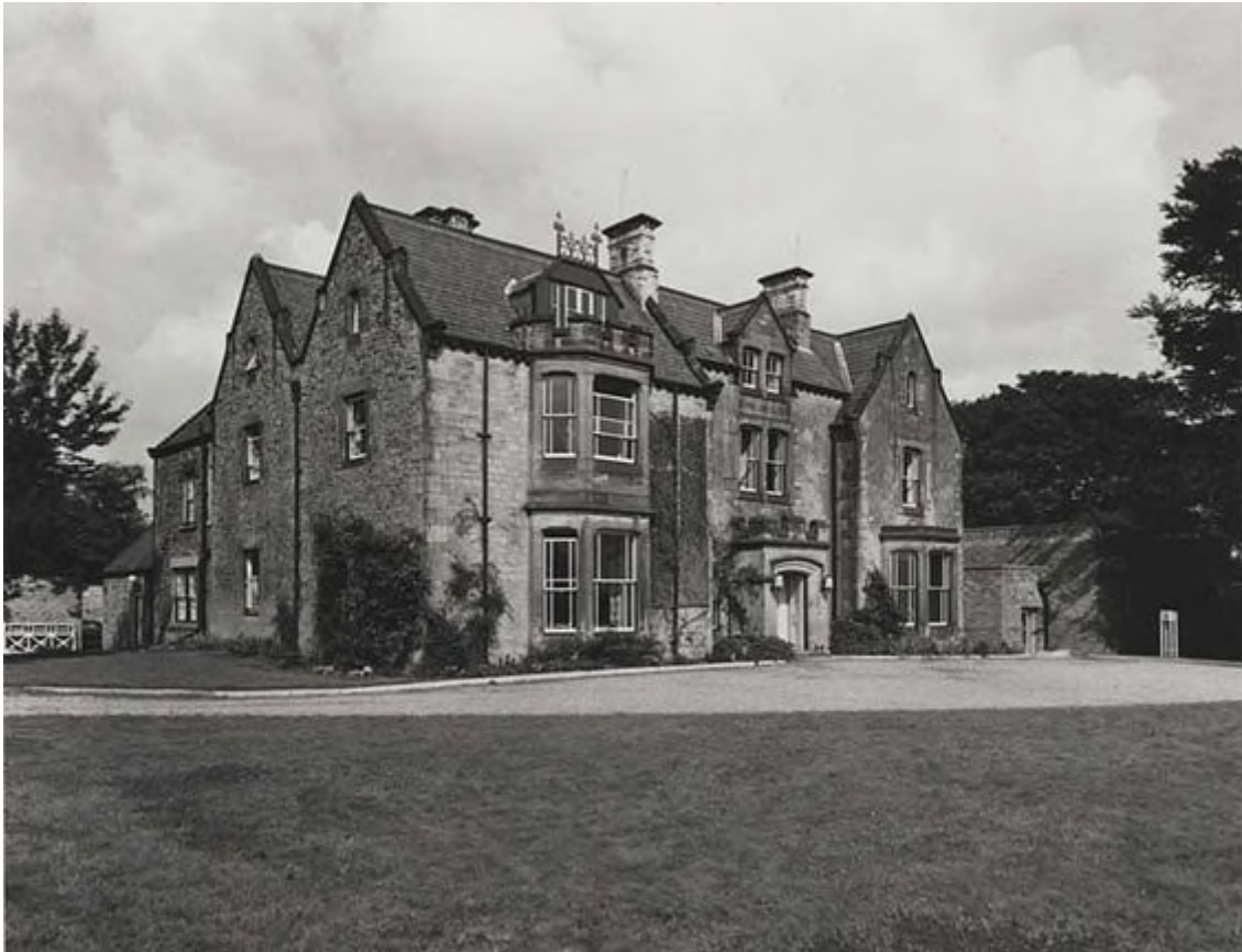
Chester-Le-Street. Newcastle Grid Control Centre (cc1958)
